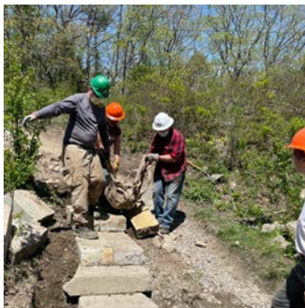
Kate Johnson, an AMC professional trail crew leader, taught the advanced group how to build stone steps at one of the four trail skill building workshops at the Fore River Sanctuary in Portland in May
